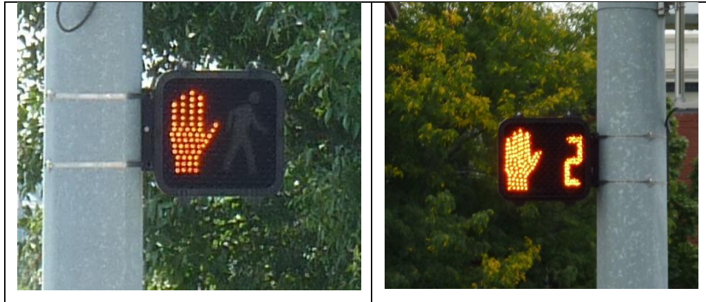
Figure 2: Traditional Pedestrian Signal (left) and Pedestrian Countdown Signal (right)
